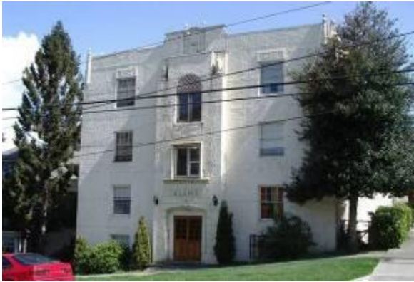
The historic Alamo Apartments on Maple Street and Garden Street. Photo courtesy Bert Monroe.
